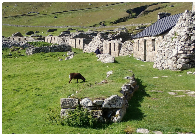
Deserted and dilapidated – what is left of the main street of St Kilda. The house on the right appears to be inhabited by visitors, it has a roof.
