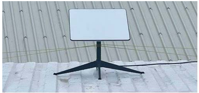
Starlink satellite antenna fixed to a Tristan rooftop
